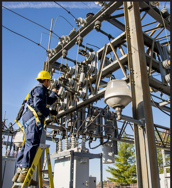
Staff Sgt. Manoj Williams, a 375th Civil Engineering Squadron electrical systems craftsman, greases framework knife blades and tightens loose conductor connections at Scott Air Force Base, Ill. (U.S. Air Force photo by Airman Daniel Garcia)
